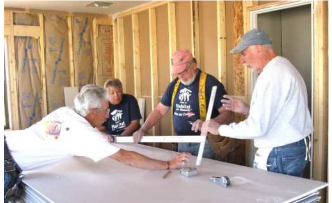
Drywalling at the Gallegos house
