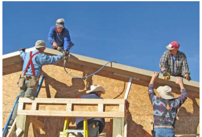
View of the soffit on the Balderrama's house
